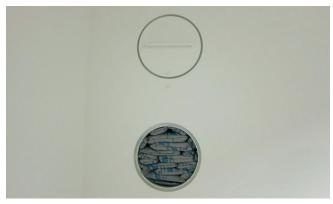
HVS cable fire protection partition (scenographic); on top: with cover; bottom: filled with fire-stop pads, without cables
