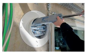
Installation of HVS fire-stop pads with the help of the assembly plate
