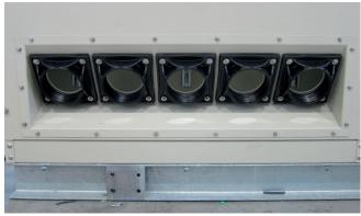
According to the requirements the appropriate sealing covers can be fixed on the fl anges HSI 150-DF. The positioning of the cable entries was done according to customer requirements. Due to the angular installation of the fl anges the ideal laying of cables was granted including compliance to the minimum bending radius.
