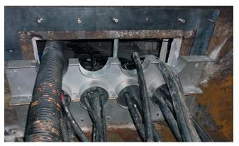
Adhesive bonding of the flat seal via Sikaflex sealing compound.
