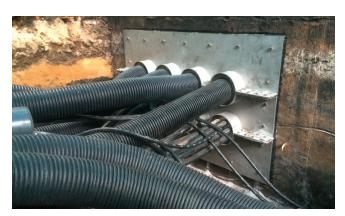
Ready installed flange plate with cable and pipe penetrations.
