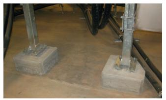
Concrete footings installed to raise steel works off water level
