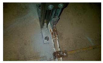
Passive fire protection materials washed out of the penetrations and water damaged the steel footings
