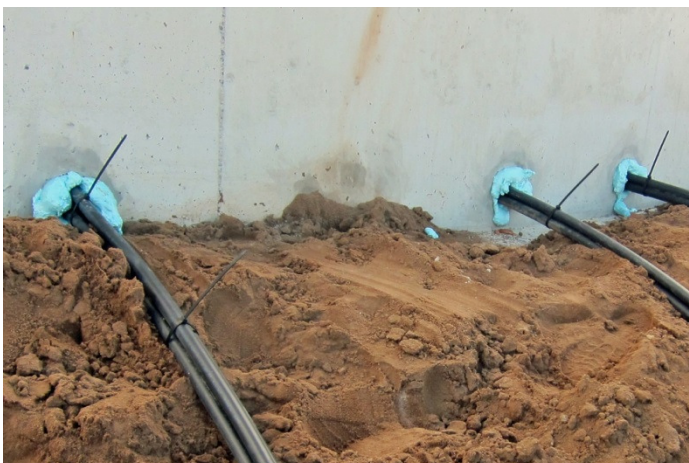
Unprofessional sealing of power cables on the outside of the foundations
