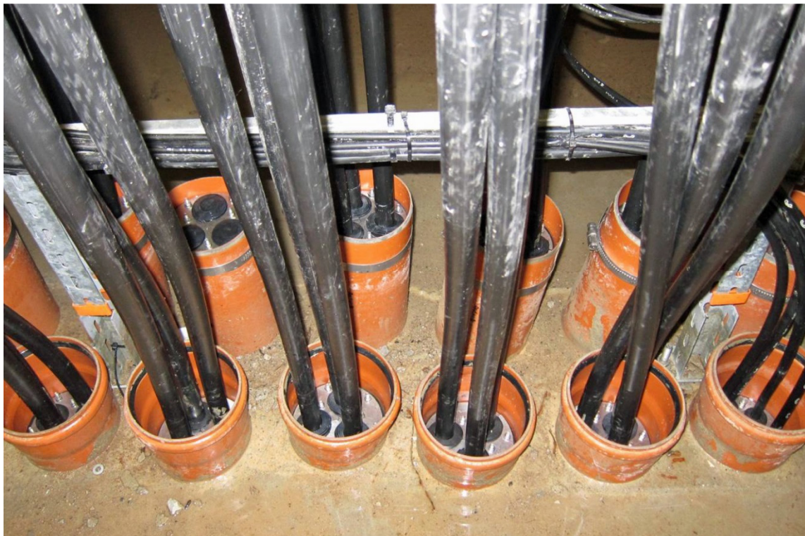
Renovation using standardized press seals with segment rings
