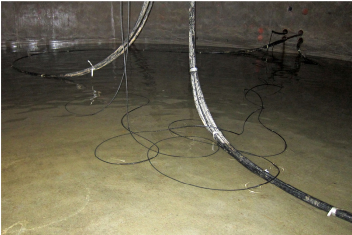
Ingress of water in the foundations of a wind turbine
