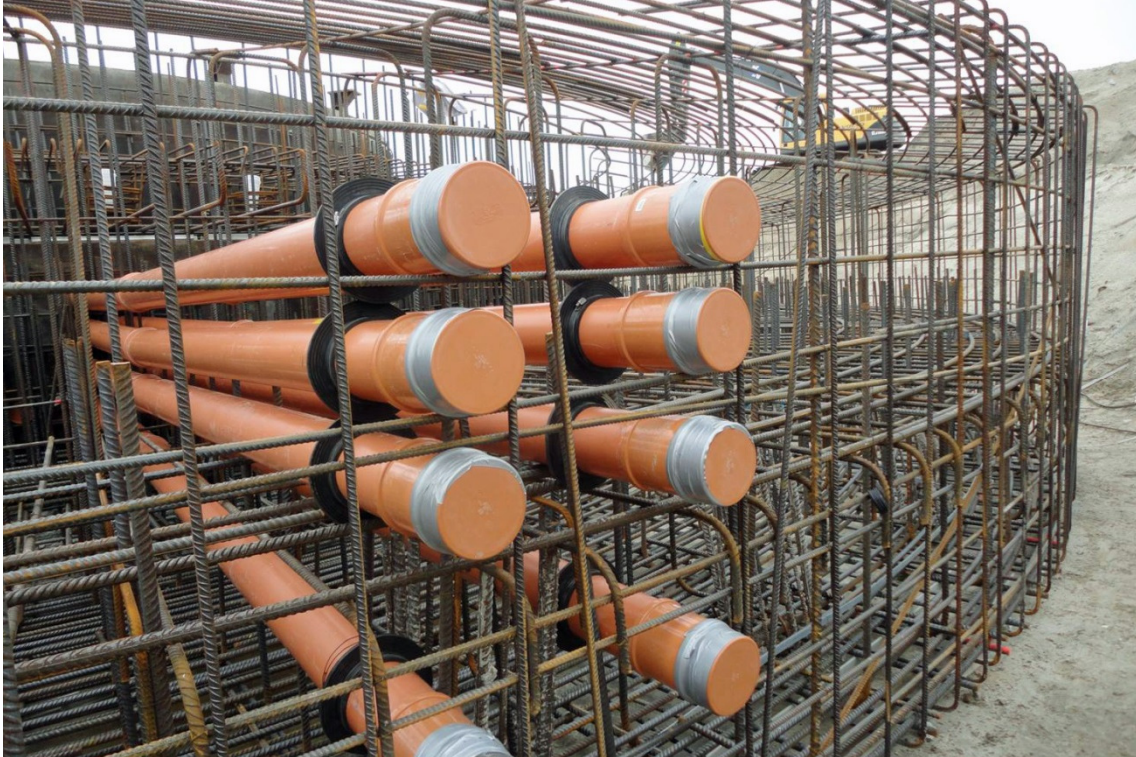
Wastewater pipes with water barrier placed in the reinforcement of the foundations
