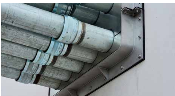
Stainless steel flange split for subsequent dowelling
