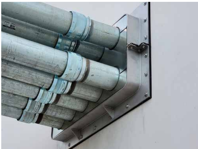
Stainless steel flange split for subsequent dowelling
