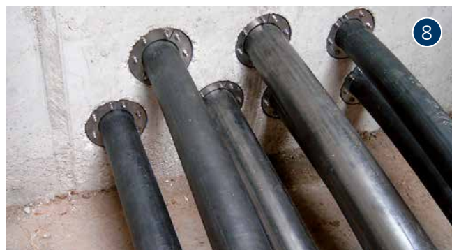
HRD press seals installed
