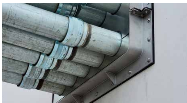
Stainless steel flange split for subsequent dowelling
