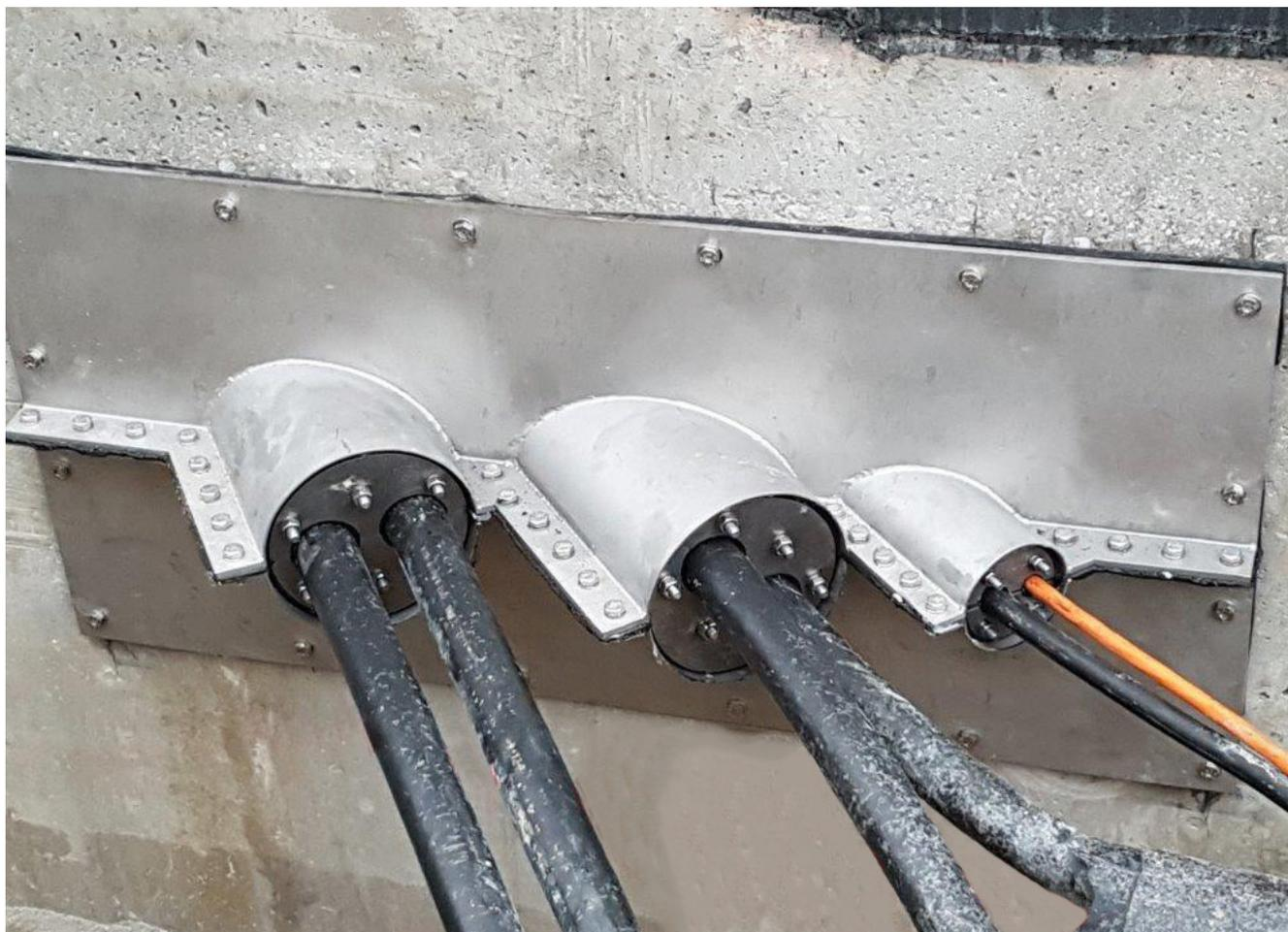
KABELSKA UVODNICA S PRIRUBNICOM OD NEHRĐAJUĆEG ČELIKA HRD2X150-
