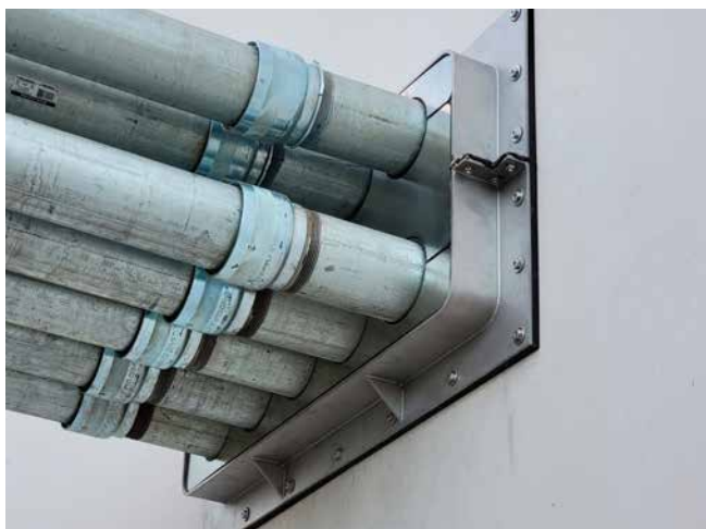
Stainless steel flange split for subsequent dowelling
