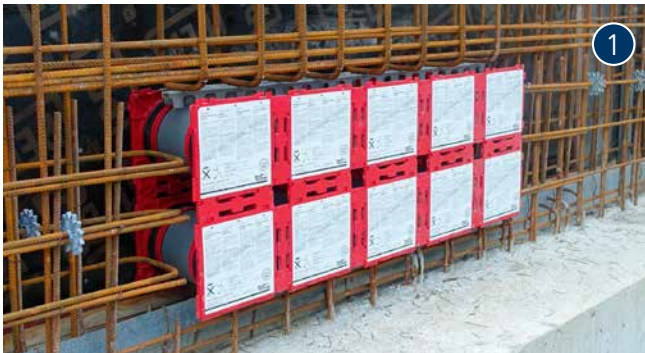
double wall insert HSI150 K2 before concreting
