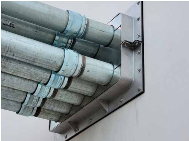
Stainless steel flange split for subsequent dowelling
