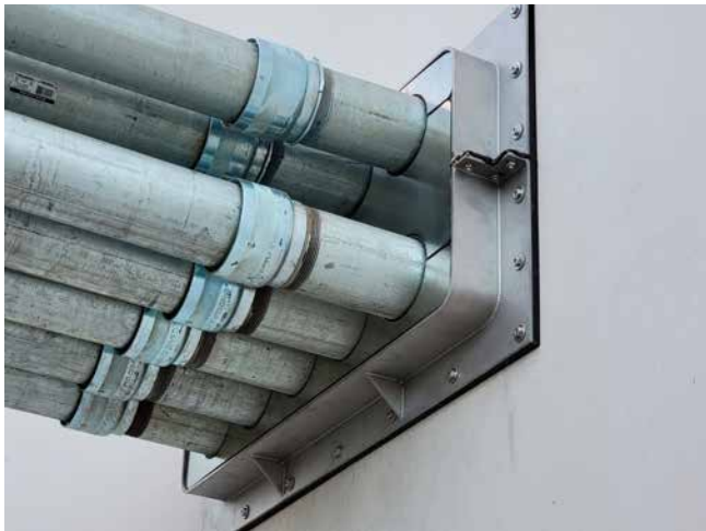
Stainless steel flange split for subsequent dowelling
