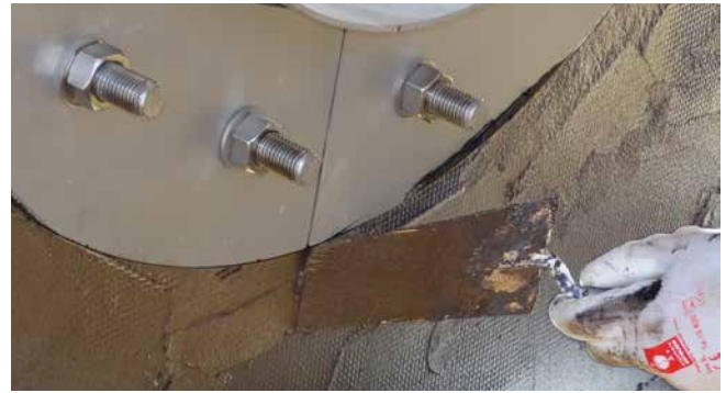
FLFE 1x200/X stainless steel design with connection to PMBC by means of fleece inlay
