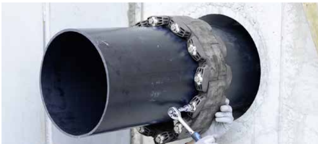
GKD400 – tightening of segments
