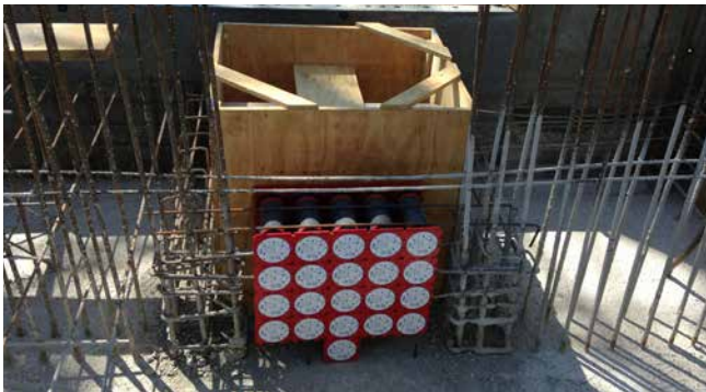
assembly of double wall insert HSI90 before concreting
