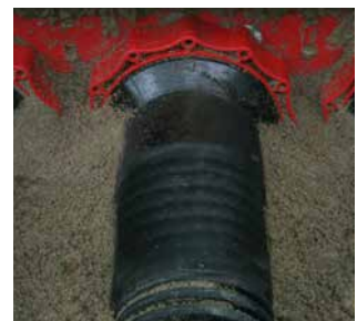
connection of corrugated pipes with cold shrink sleeves HSI150 D1x110 KS WR
