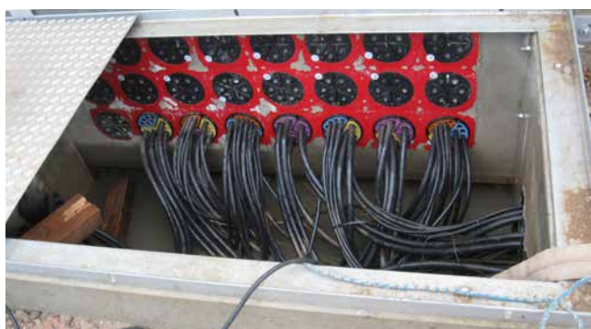
HSI150 – wall inserts fitted with SEGMENTO sealing for control cables in a transformer house
