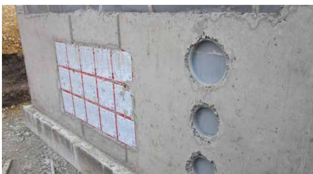
ZVR150 and ZVR200 set in concrete next to HSI150
