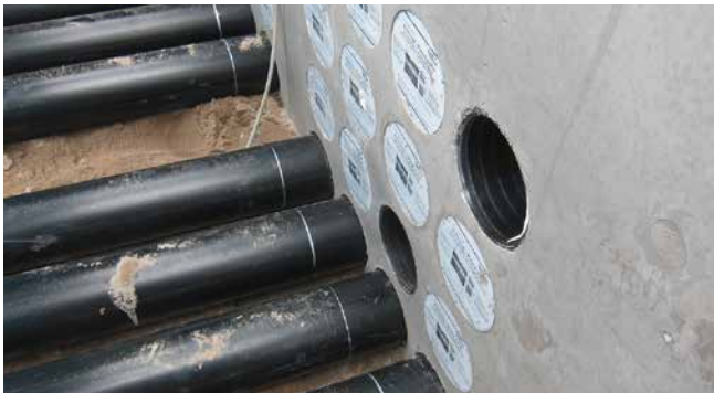
HSI150 GSM installed
