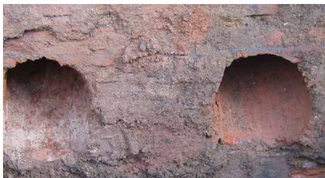
slanted core drill in porous wall
