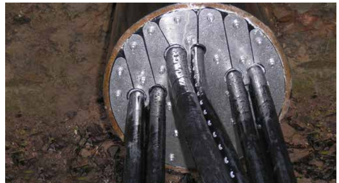
HRD200 G b30 installed in a steel pipe
