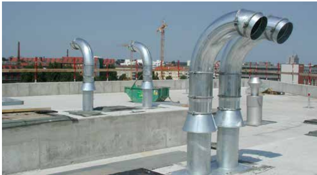
installed SHD200 before laying of cables
