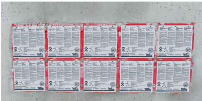
double wall insert HSI150 as block assembly
