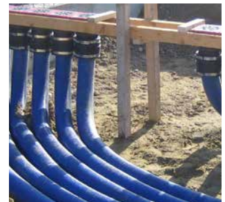
side by side arrangement 2x KES150 MA ZVR150/500 on the installation fixture KES FUBO-FIX AV
