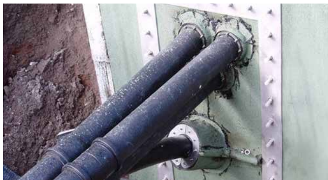
split fixed/loose flange according to DIN 18533
