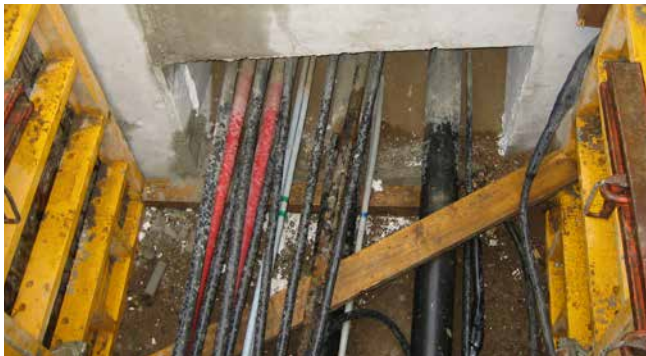
existing rectangular recess – has to be subsequently sealed
