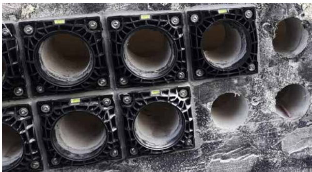
core drill and dowel holes prepared for installation of HSI150 DFK
