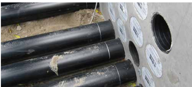
HSI150 GSM Varia applied as a block
