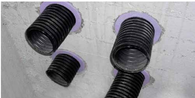
view of inside of building (insulation ring)
