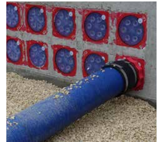
pressure-tight connection to HSI150 wall inserts
