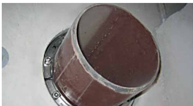
HSD200 1x160 b40 A2/EPDM55 – drainage SML pipe
