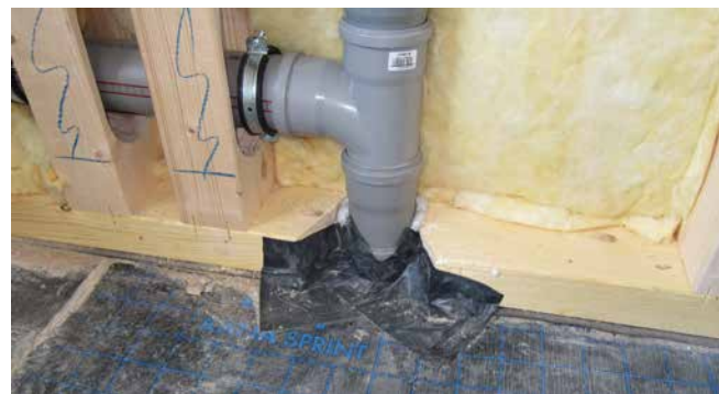
difficulty: integration of vapour barrier foil
