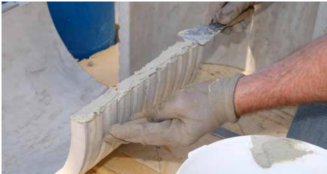
FZRG350/300 with levelling compound from installation set MSET FZRG
