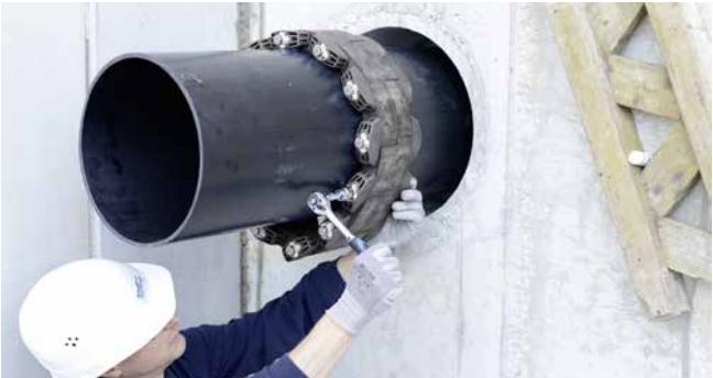
GKD400 - tightening of segments
