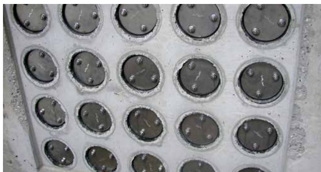
FZR100/240 - pipe section sealing
