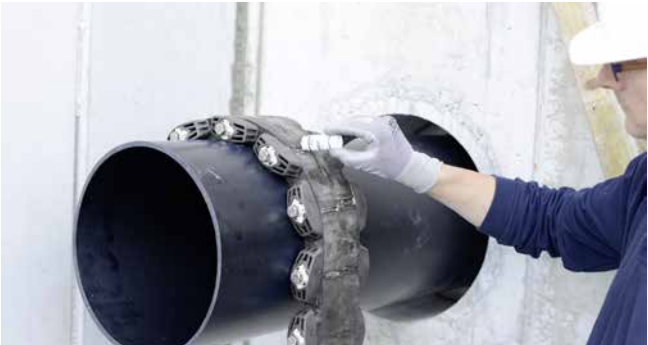
GKD400 - installation preparation with lubricant GM
