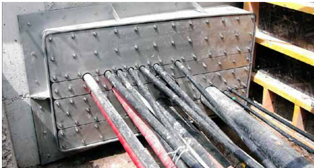
rectangular split flange for several cable penetrations
