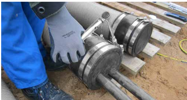
pressure-tight connection of spiral hose Hateflex14090 to wall insert HSI90 and end stop for the cable duct
