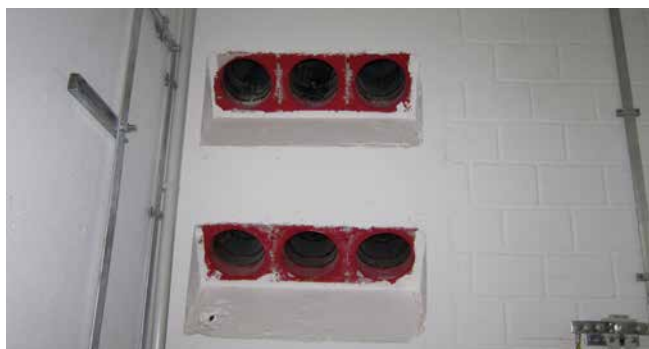
section 2x HSI150 1xZ K2 S45°/X double wall insert
