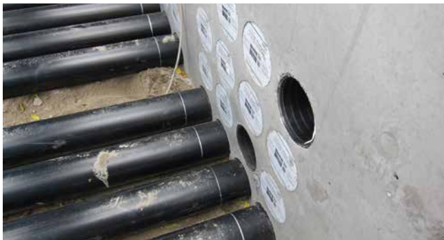
HSI150 GSM Varia applied as a block
