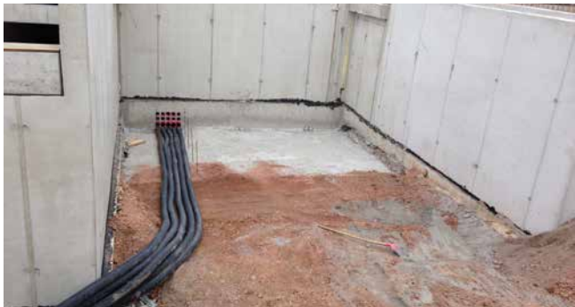
connection of corrugated ducts HSI90 D1x75 KS WR
