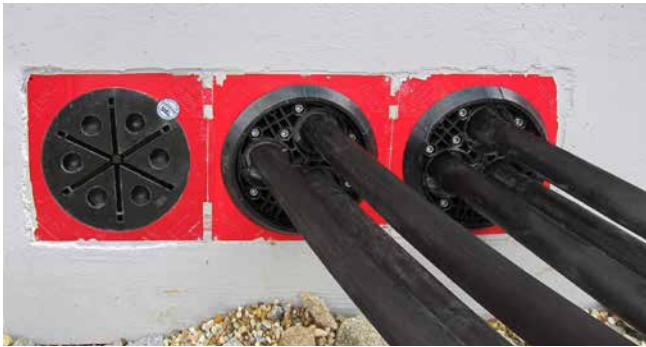
various installation stages for HSI150 DG 3x24-54
