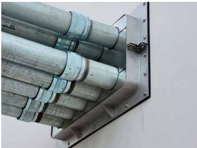
Stainless steel flange split for subsequent dowelling
