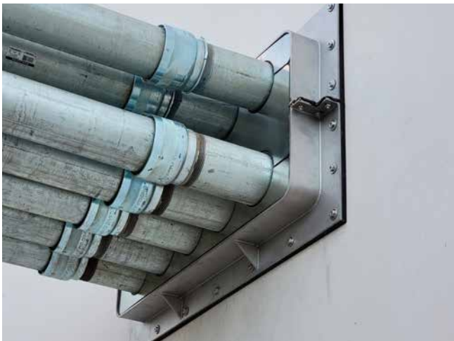
Stainless steel flange split for subsequent dowelling
