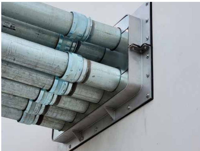
Stainless steel flange split for subsequent dowelling
