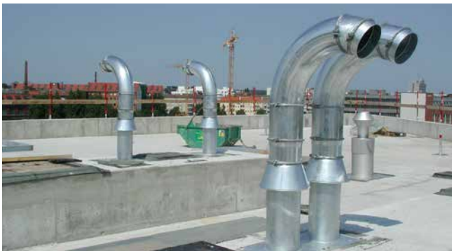
installed SHD200 before laying of cables
