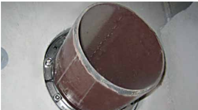
HSD200 1x160 b40 A2/EPDM55 – drainage SML pipe
