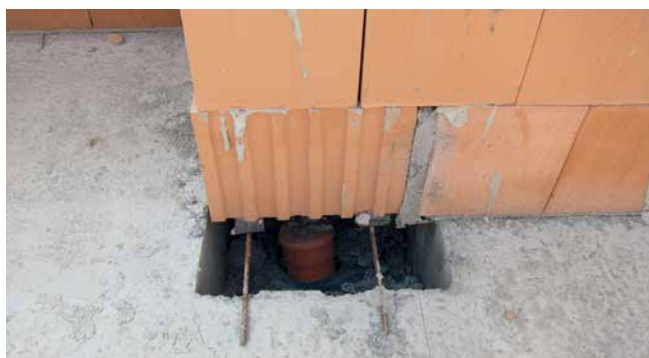
difficulty: retrofit gas-tight and vapour-proof sealing
