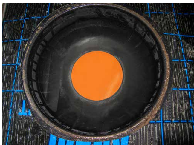
easy integration of the vapour barrier using the adhesive ribbon
