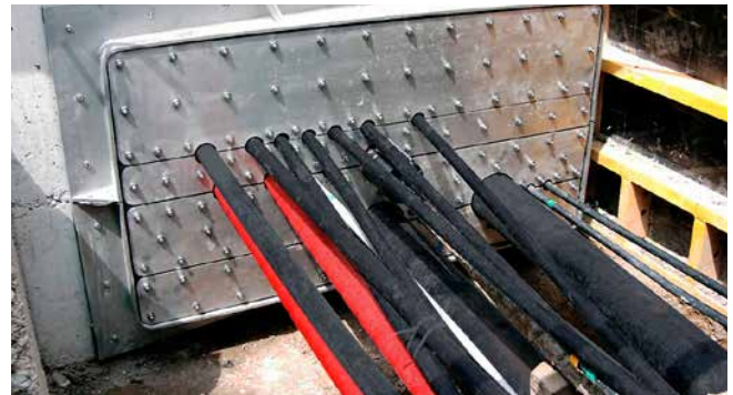
split rectangular flange with multiple cables
