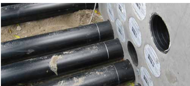
HSI150 GSM Varia applied as a block
