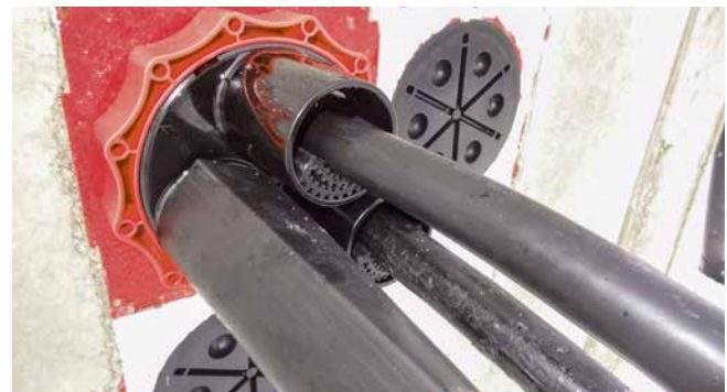
centring tape in system cover plugs of HSI150 D3x58 WS
