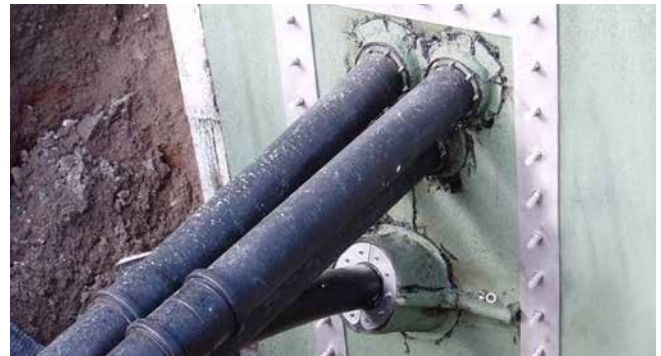
split fixed/loose flange according to DIN 18533
