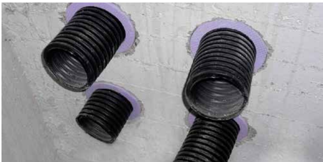
view of inside of building (insulation ring)
