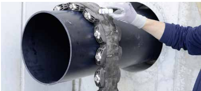
GKD400 – installation preparation with lubricant GM
