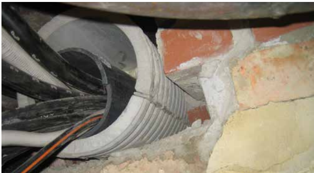
FZRG150/350 – refurbishment in masonry
