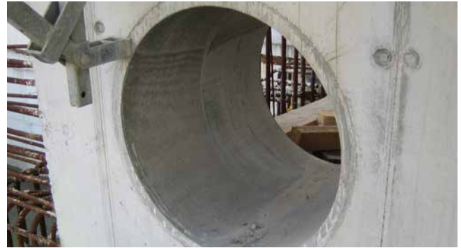
FZR400/300 – installation in water treatment plant
