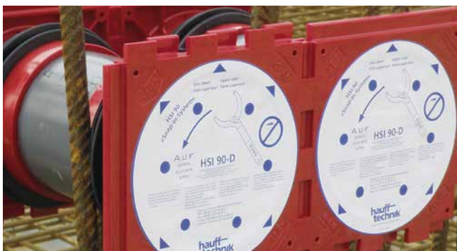
double wall insert HSI90 as block used in formwork
