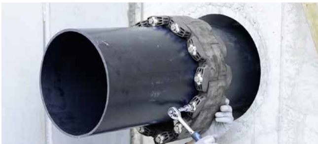
GKD400 – tightening of segments
