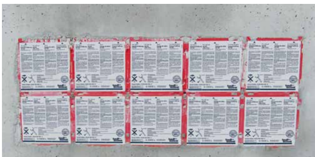
double wall insert HSI150 as block assembly
