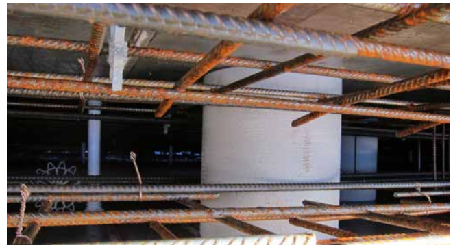
ZVR200/300 fixed in formwork
