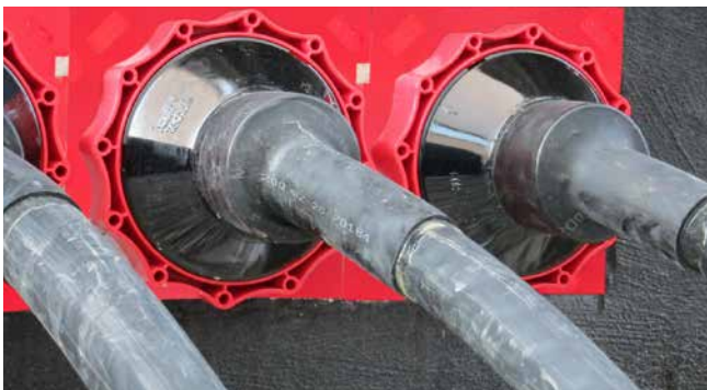
station entry: low-voltage cable sealed with HSI150 D1x80 WS
