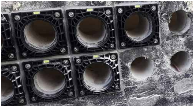
core drill and dowel holes
