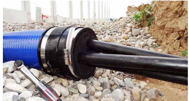
sealing in soil at the end of spiral hose Hateflex14150 with the sealing set KES150 MA WE 160 SG 3x22-58 SET
