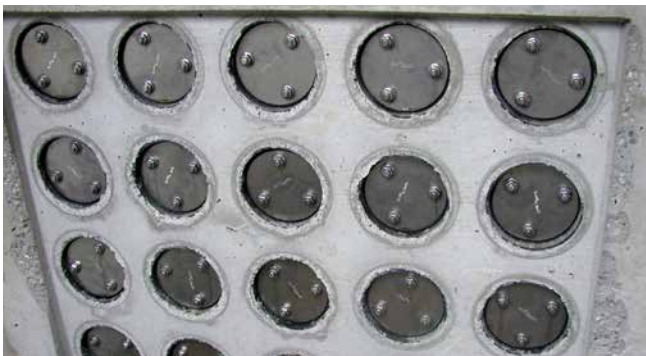
FZR100/240 – pipe section sealing
