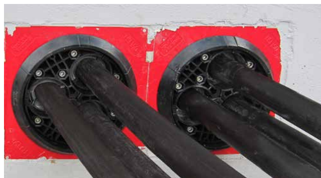
various installation stages for HSI150 DG 3x24-54
