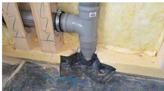
difficulty: integration of vapour barrier foil
