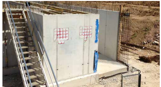
HSI90 after concreting: empty ducts are installed subsequently
