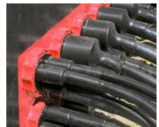
station entry: low-voltage cable sealed HSI90 D1x75 WS and HSI90 D3x32 WS
