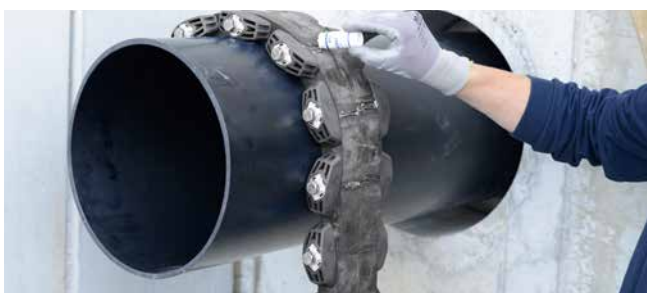
GKD400 – installation preparation with lubricant GM
