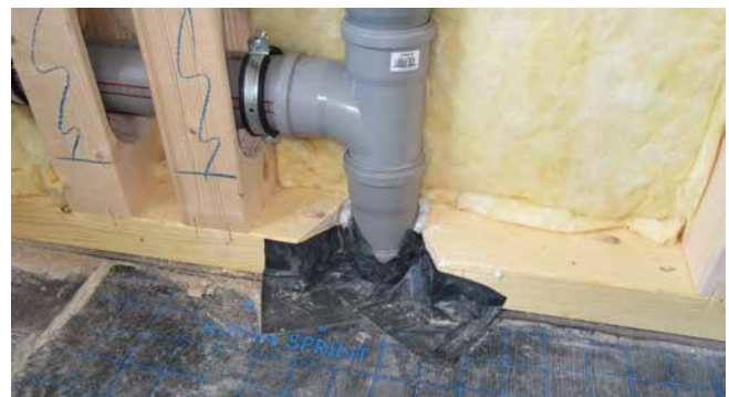
difficulty: integration of vapour barrier foil
