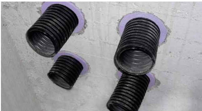
view of inside of building (insulation ring)
