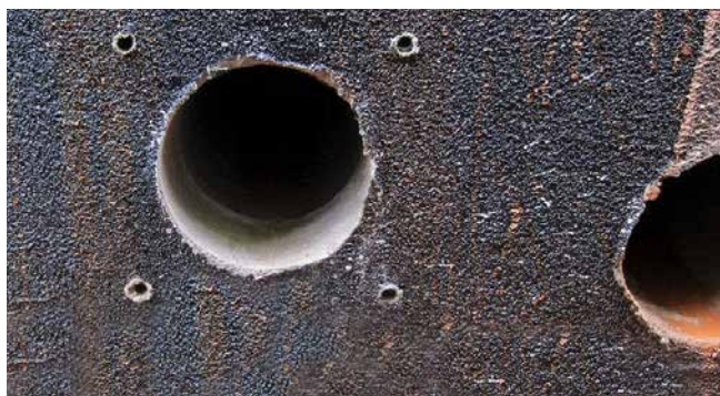
core drill and dowel holes
